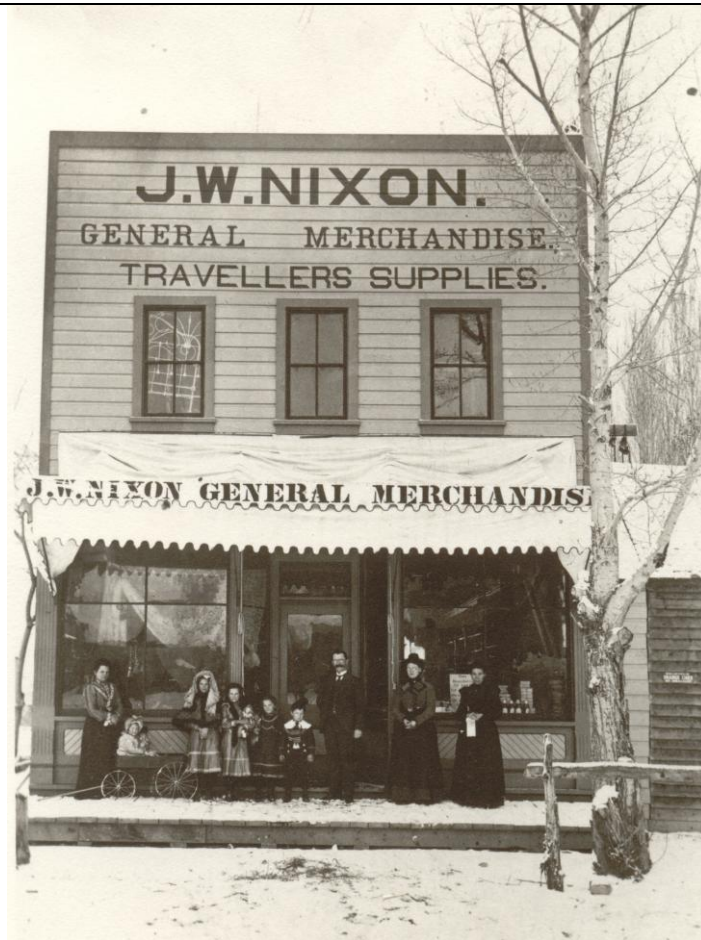
J. W. Nixon Store before additions:
