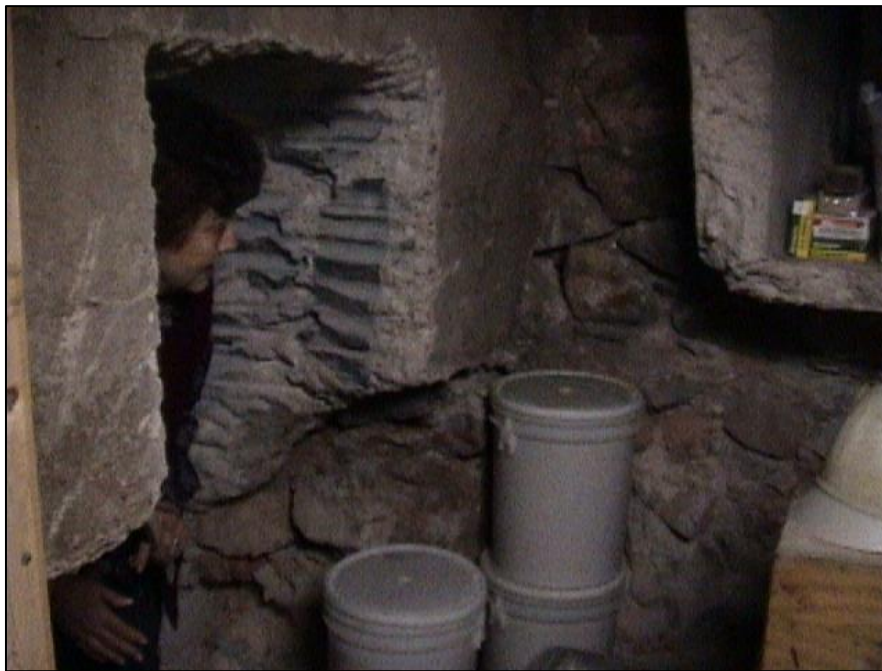
James W. Nixon I Home basement, St George, Utah, ca. 2000
