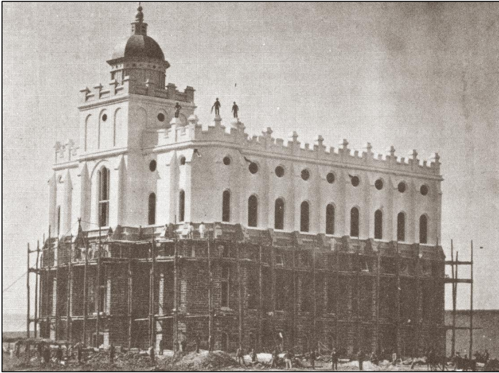
St. George Temple under construction
